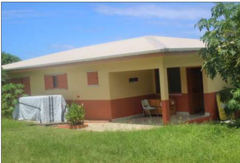
The Provincial Disaster Office Building in Isangel, Tafea Province
